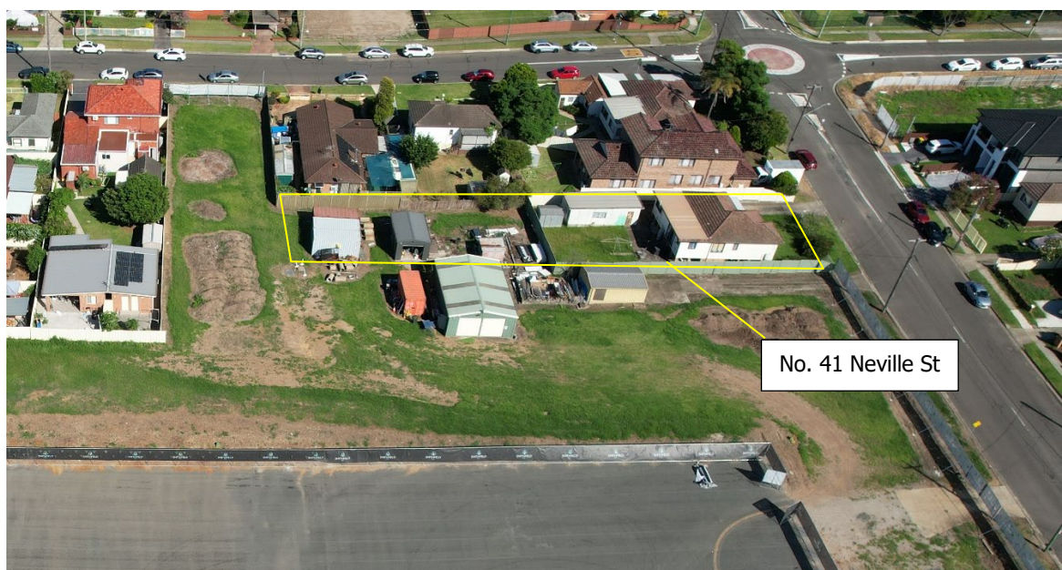
Plate 24: Aerial view of the 41 Neville Street, looking west (source: Benson McCormack Architects).
