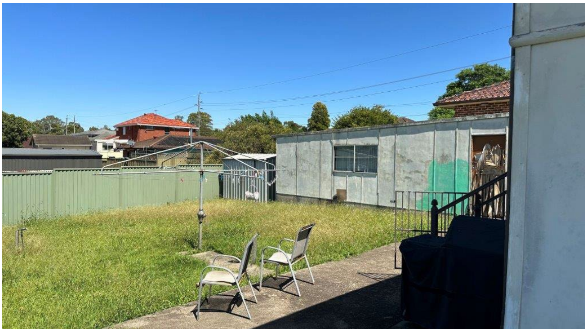
Plate 26: View towards the south-west showing the rear yard and sheds of the dwelling on No. 41 Neville Street.
