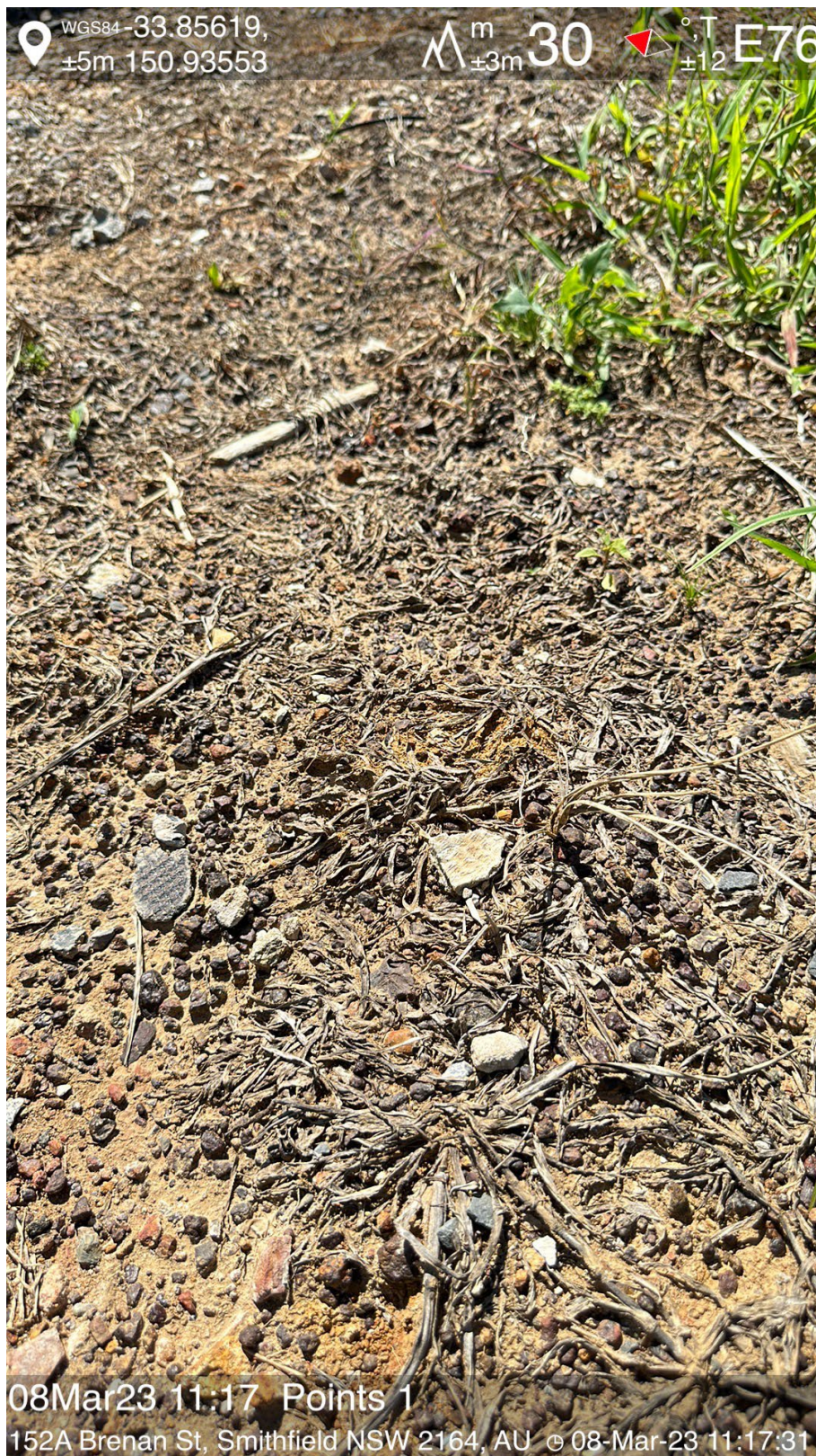
Plate 50: Example of potential ACM observed on the surface of 152a Brenan Street.
