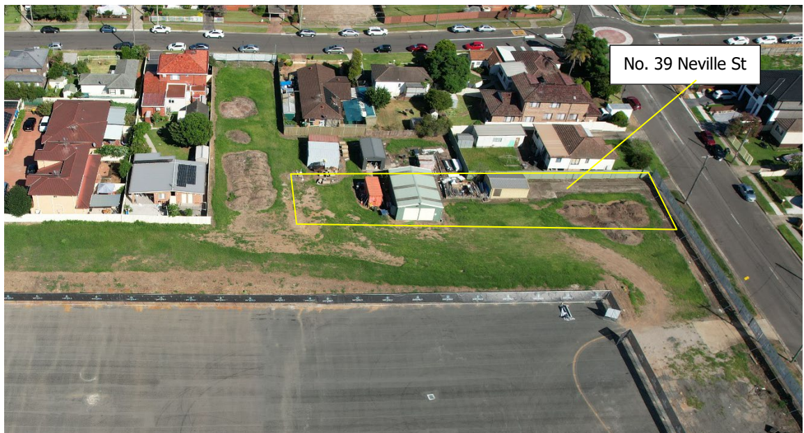
Plate 19: Aerial view of the 39 Neville Street, looking west (source: Benson McCormack Architects).
