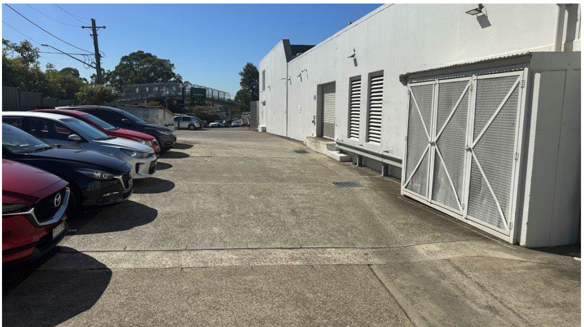
Plate 3: View towards the east along the northern side of the RSL Club Building. Driveway and loading dock.
