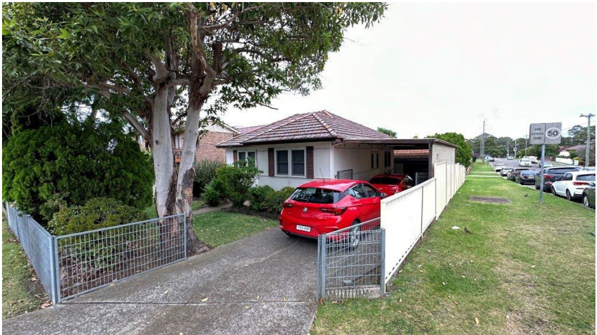
Plate 34: View to the south-east showing the front of No. 45 Neville Street.
