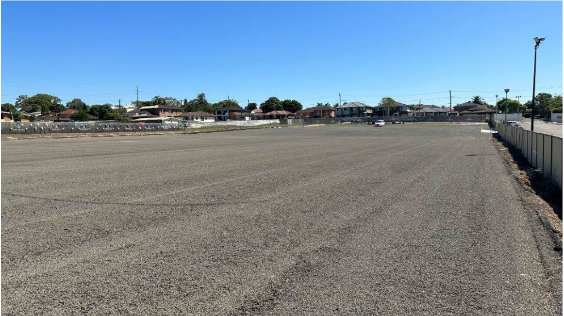
Plate 10: View towards the north across the recently constructed carpark.
