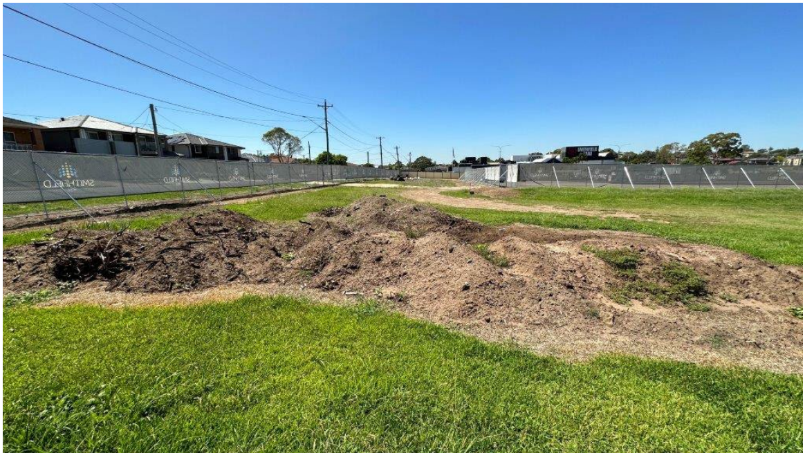
Plate 22: View towards the east showing the soil stockpiles on the northern end of No. 39 Neville Street.
