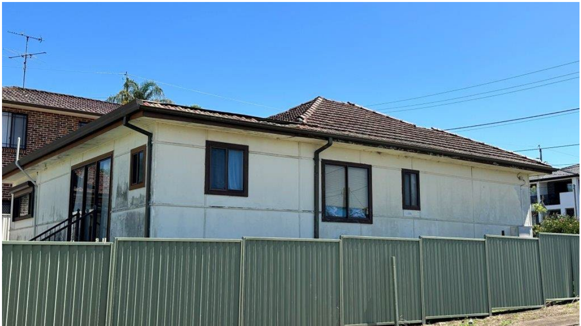
Plate 25: View towards the north-west showing the dwelling at the northern end of No. 41 Neville Street.
